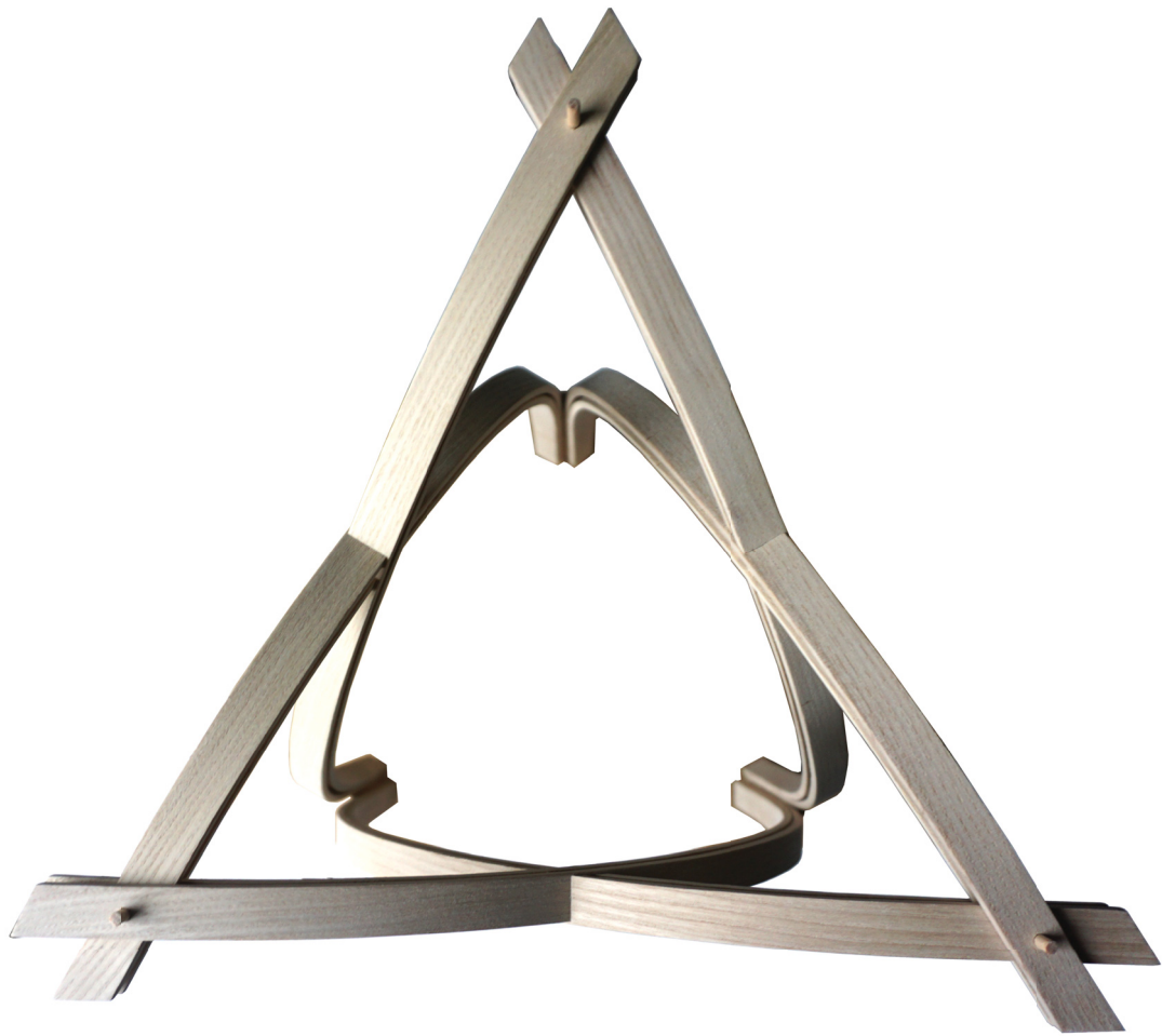
Top view of Bent Wood Pavilion, using a triangular grid of identical, bent components.
