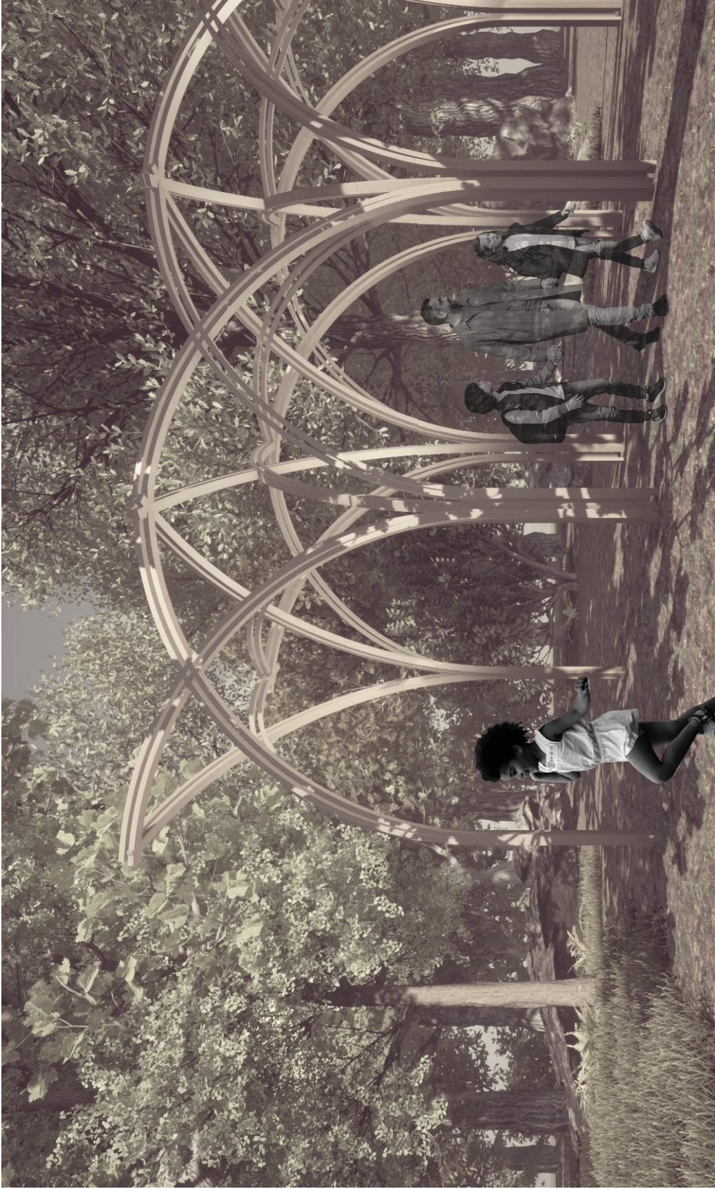
Rendering of Bent Wood Pavilion expanded into a larger configuration along a triangular grid.
