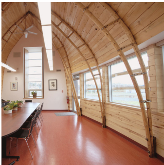
Bentwood trusses in Pictou Landing Health Center (Kroeker n.d.)
