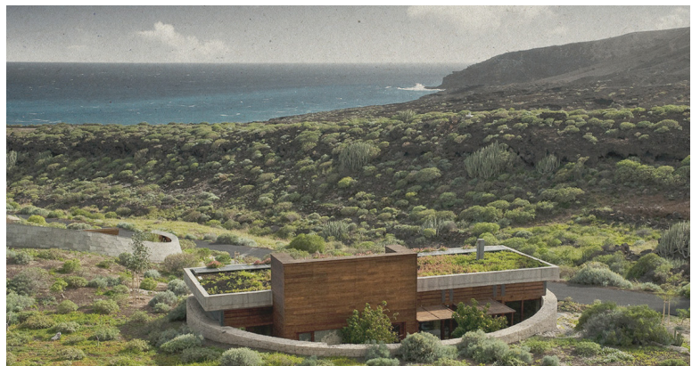
A bioclimatic dwelling in Tenerife by Ruiz Larrea y Asociados. Notice how it conveys and integrates with nature through form and material. (Ruiz Larrea y Asociados 2000)
