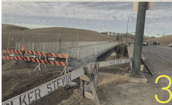
3 New pedestrian infrastructure crossing the highway north/ south.
