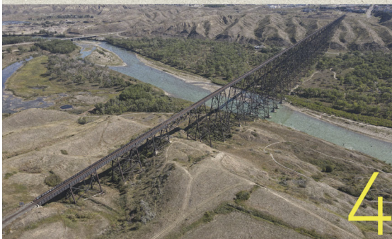
4 The Lethbridge Viaduct. (Malefant 2021b)
