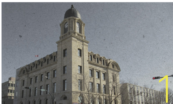
Lethbridge post office. (Bencito the Traveller 2012)
