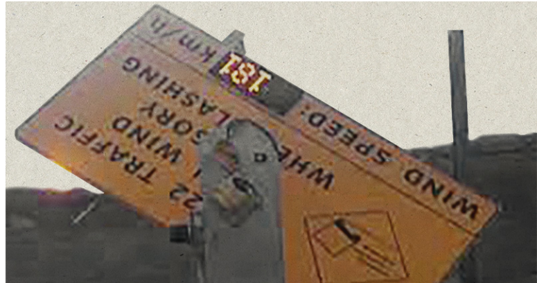
Damaged wind speed sign one hour outside of Lethbridge after a chinook gust of clocked at 181 km/hr. (Houck 2018)
