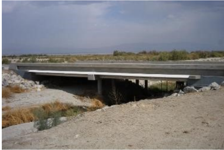
Figure 2-37. Kings Stormwater Channel Bridge (HPWREN, UCSD/CalTrans)
