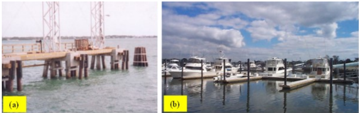
Figure 2-39. (a) Fender piles and dauphin clusters in Naval Station Ingleside Project; (b) Structural piles in Belmar Municipal Marina Project (Fam et al. 2003)
