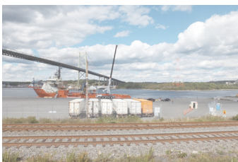
Mackay Bridge and port, Halifax
