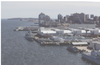
View looking south of naval infilling, from the Macdonald Bridge
