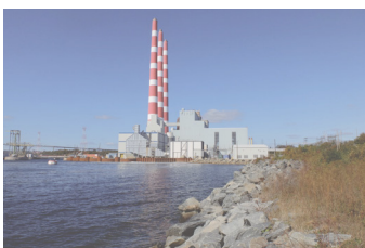
Looking north to energy station, Dartmouth
