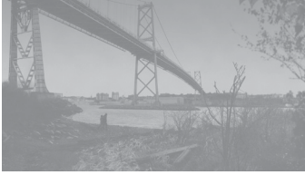
Under the Macdonald Bridge, montage
