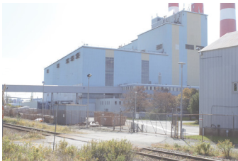
Looking south toward the water from behind Tufts Cove energy station
