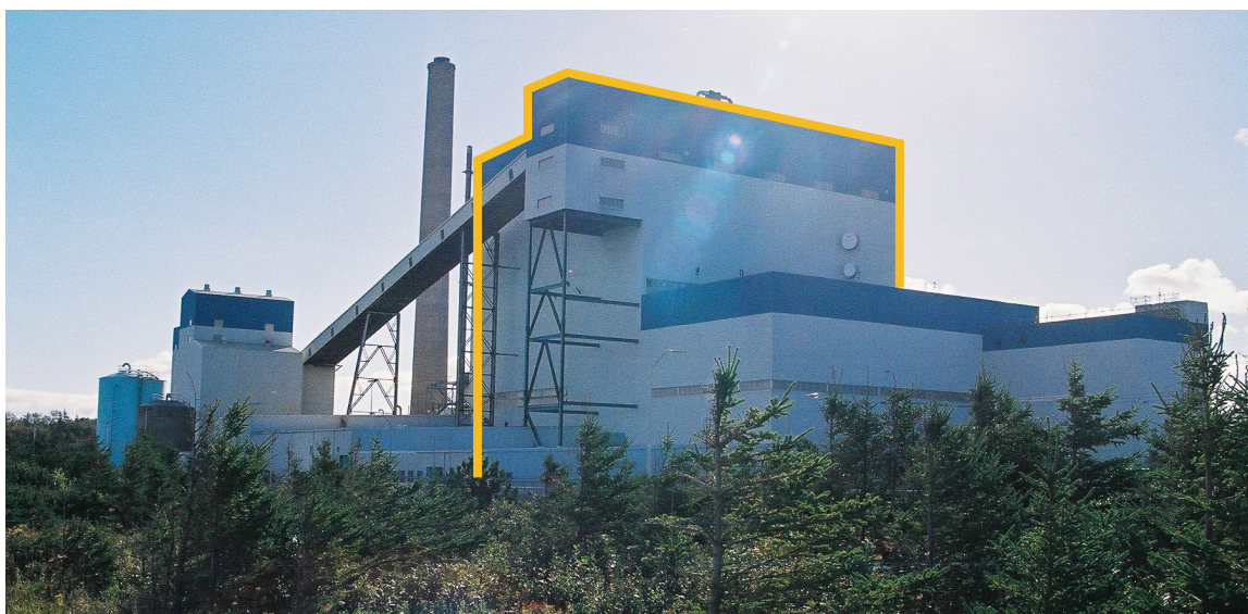
Image from the northwest edge of the site, looking at the plant from the public beach.
