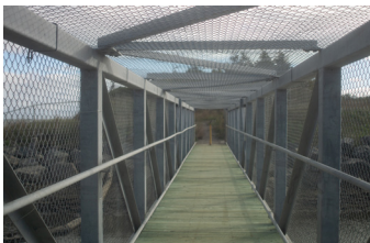
Interior view of walkway
