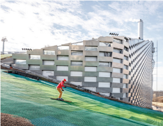
Rooftop Ski Trail (Hjortshoj 2019)
