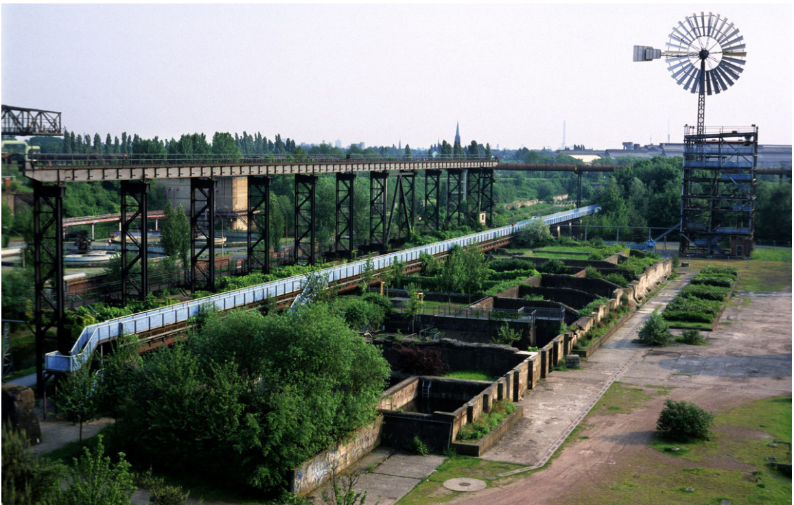
View of the Landschaftspark Ore Bunkers which was a highly toxic region of the site where soil and planting was introduced to begin remediation. (Latz 2002)
