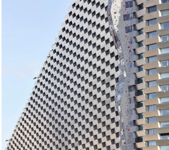
Outdoor Climbing Wall (Hufton + Crow 2020)
