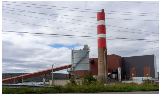
Point Tupper Generating Station - 154MW Opened in 1973
