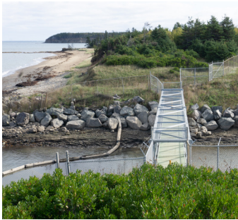
Enclosed public walkway allows the public to continue to the eastern part of the beach past the plant's water output into the ocean.
