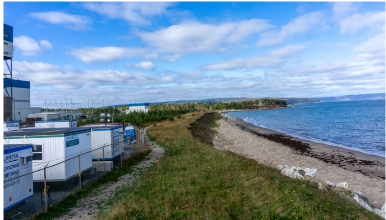
View of public path and beach adjacent to plant.
