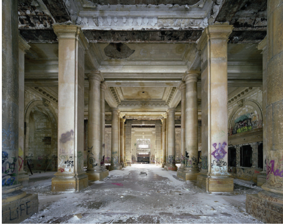
The corridor linking the atrium and the concourse as it exists today (Marchand and Meffre 2013)
