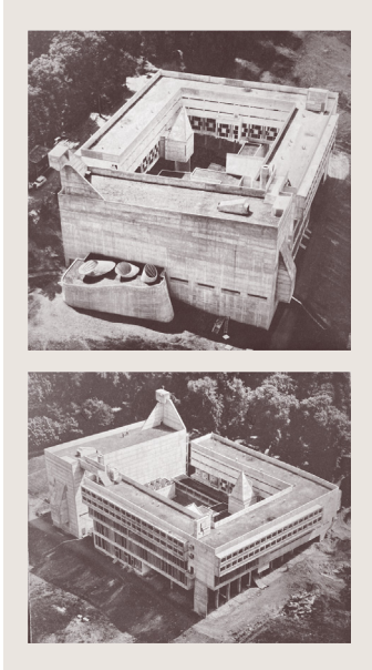
Aerial view of La Tourette from the north (top) and the west (bottom), 1966; photographs by Bernhard Moosbrugger (Henze and Moosbrugger 1966, 66-67)
