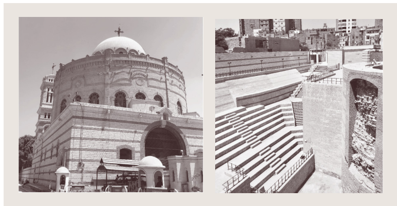
Left: photo of St. George’s Church in Old Cairo located within the Fortress of Babylon (right), showing the exterior use of brick 2019.
