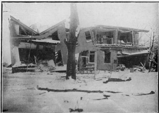
All that is left of two homes in the Richmond section.
