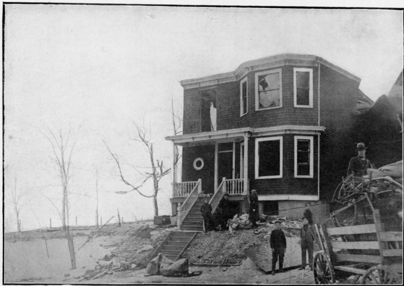
This house is situated more than a mile from the scene of the explosion, but the interior was completely wrecked and the furniture was blown out on the street
