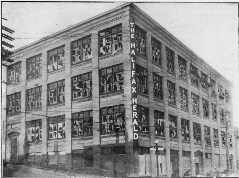
THE HOME OF THE HALIFAX HERALD AND THE EVENING MAIL AFTER THE EXPLOSION. The Herald building is situated more than two miles from the scene of the disaster, and so great was the explosion that every pane of glass in the building was shattered. On the north and west sides (not shown in the picture) the greatest damage was caused, frames and glass being blown in on the presses and other parts of the plant.
