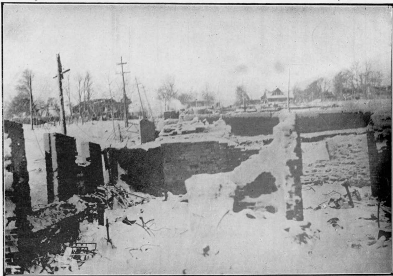
This is a scene at Richmond and shows how completely the buildings in that section were demolished.
