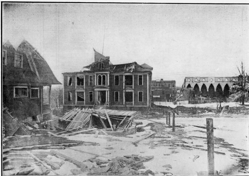
A view of the wrecked St. Joseph's School, with the ruins of St. Joseph's Church showing in the rear.
