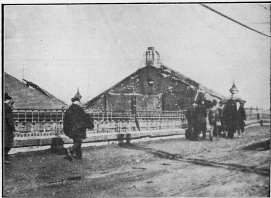
This view is looking down on the roof of North Street Station and shows how that building was battered up.
