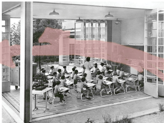
Class pavilion in L'École de Pleine Air with three opened walls (Lods 1936)
