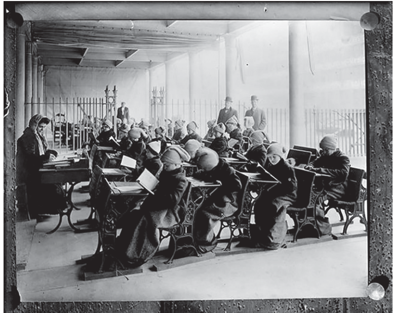
A set of columns allow the walls to be open to the exterior in an open air school in New York, 1910. (Riis 1910)
