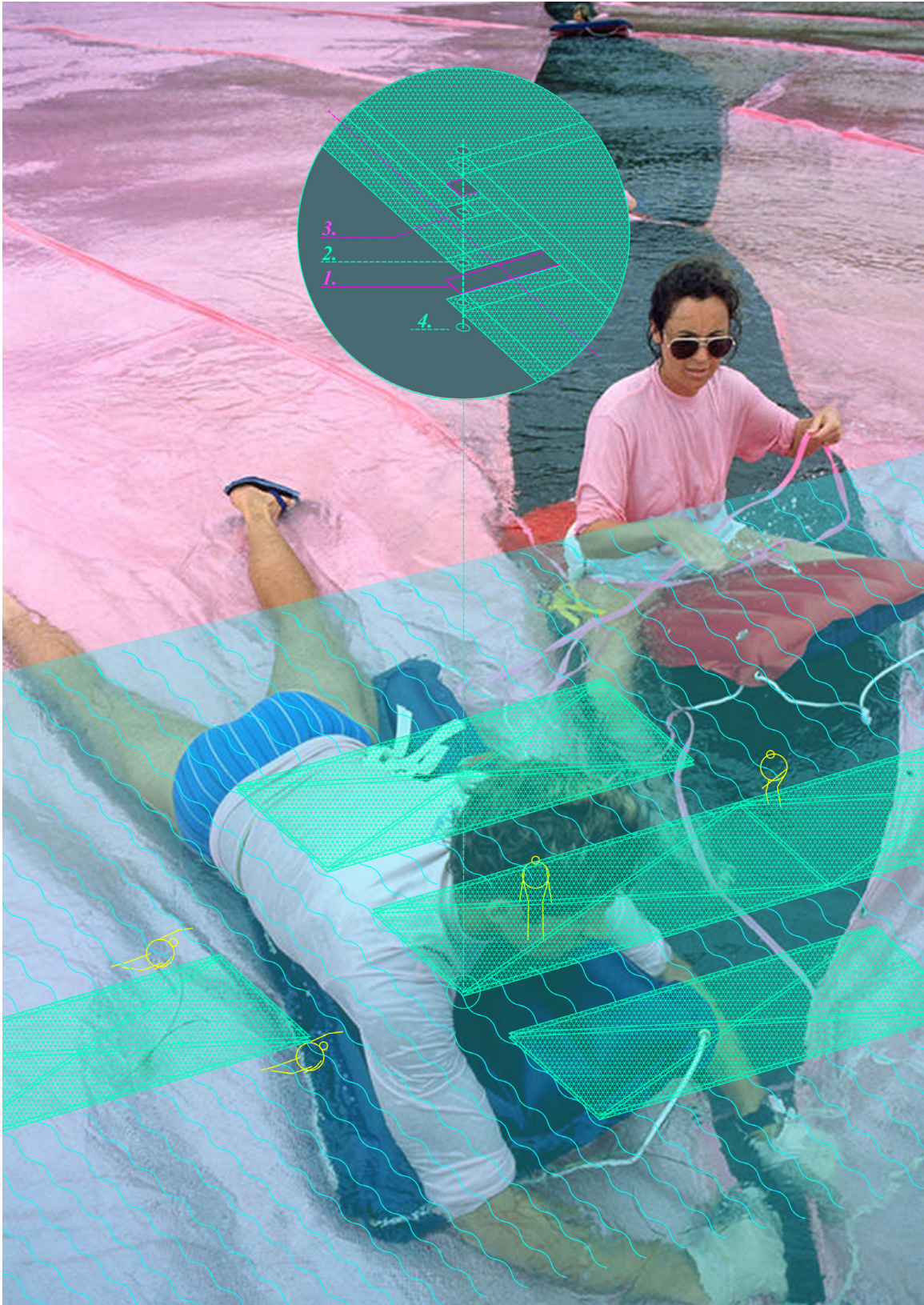
020 SMOG: assembly 1. smog (heat) activated seal, 2. LX1 membrane, 3. line of smog, 4. rope system
