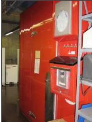
Figure 4. Outside view of a typical cold room. Source: Paula Francis, 2007.
