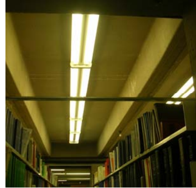
Figure 6. Uncovered T-8 32W bulbs. This setup was also found covered in other parts of the Killam library
