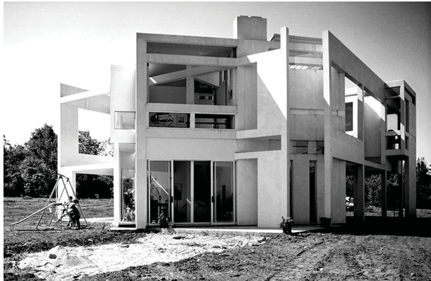
Eisenman Architects, "Physical Model" of House III in Lakeville, Connecticut, 1969-1971; photograph from Eisenman Architects' website.
