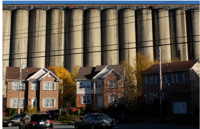
Photo showing off-scale height of the silos' body compared to the surrounding context
