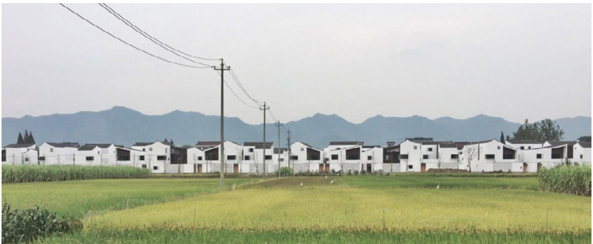
Dongziguan Affordable Housing for Relocalized Farmers, China, Gad Architecture Studio. From Xiyun, “Dongziguan Affordable Housing” (2017)
