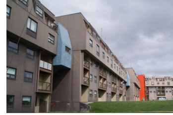
The southern interior side of the wall changes planes and has a variety of fenestration including balconies to take advantage of passive solar; photograph by Gordon Parsons
