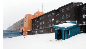
The north and west side of Fermont's Mur-Écran has few articulations and smaller amount of fenestration, photograph by Maude Chauvin
