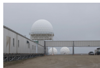
The Northern Warning System complex, Cambridge Bay, August 2018
