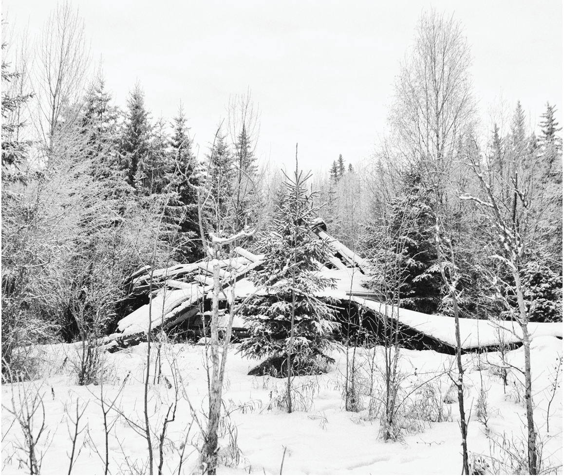
Collapsed lumber mill at Kalinowski homestead, Wildwood, Alberta, 2018.
