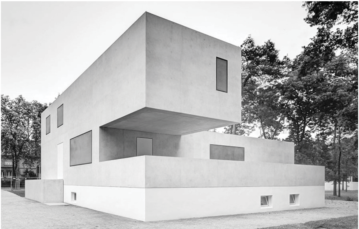
Bruno Fioretti Marquez, Masters' House , Dessau, Germany, 2014. Photo named "Gropius House" or "Directors House" from Bruno Fioretti Marquez' website.
