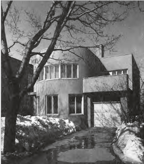
FIG. 16. PAUL LAROQUE (BEAUDRY-LEMAN) RESIDENCE, OUTREMONT, QUÉBEC, MARCEL PARIZEAU, 1936-1937. | COUTURIER, MARCEL PARIZEAU ARCHITECT
