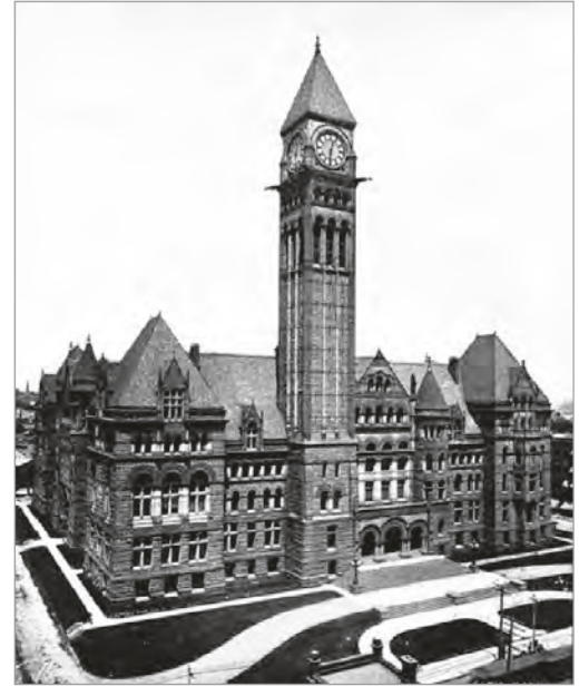
FIG. 25. OLD TORONTO CITY HALL, TORONTO, ONTARIO, E.J. LENNOX, 1889-1899. | CITY OF TORONTO ARCHIVES, SC587-19.
