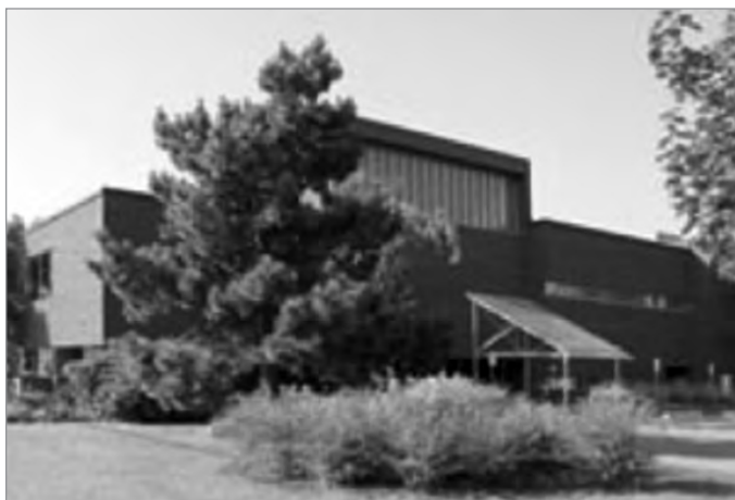
FIG. 22. RICHVIEW LIBRARY, ETOBICOKE, 1966. DUNLOP, WARDELL, MATSUI, AITKEN, ARCHITECTS. | TORONTO PUBLIC LIBRARY, [HTTP://WWW.TORONTOPUBLICLIBRARY.CA/DETAIL.JSP?R=LIB016], ACCESSED JUNE 30, 2017.
