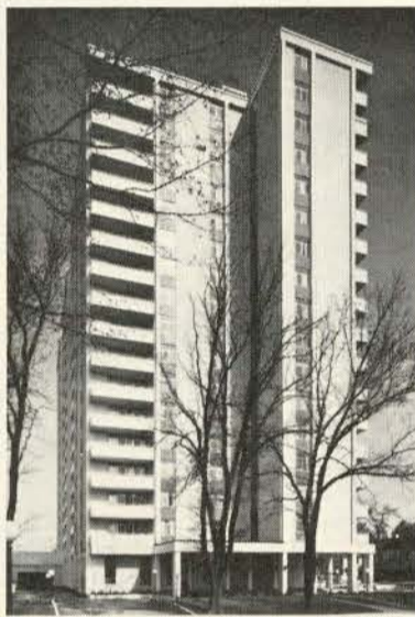
100 Queen Street North, Kitchener, Ont. Owner & Builder: Faber Construction Limited. Archt: Petroff & Jeruzalski. Cons. Struct. Engr: Alex Tobias & Associates Limited. Masonry Contr: Gottardo Contracting Company Limited. Concrete Masonry Units: Hogg Fuel & Supply Limited. Ready-Mixed Concrete: H. Boehmer & Company Limited.
