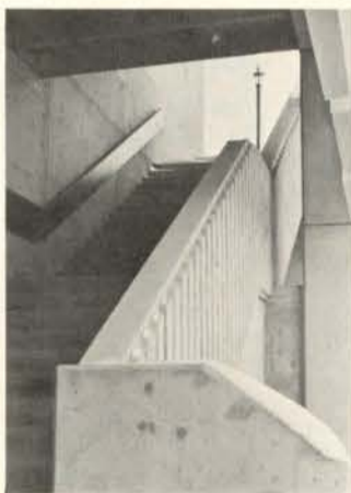
Chateau Apartments stairway from street to +15 Plaza
