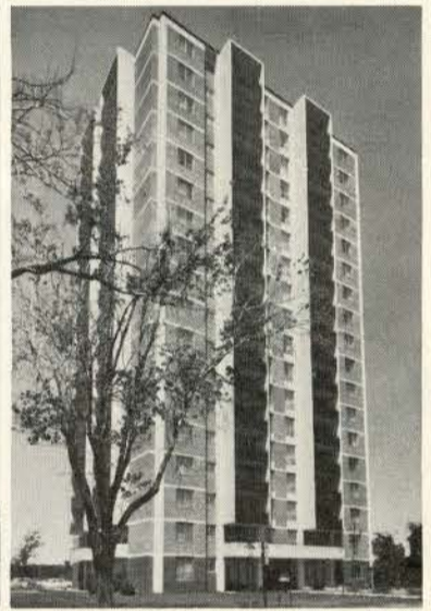
1000 Broadview Apartment Building, Toronto. Owner & Builder: Tova Developments Limited. Archt: Grozbord, King & Associates Ltd. Masonry Contr: Prime Construction Company. Concrete Blocks: Meteor Building Supplies Ltd. "Canada" Masonry Cement: Blair Supply Company Ltd.
