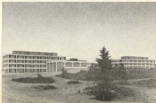
University of Saint John, Saint John, N.B. Archt: Mott, Myles and Chatwin. Gen. Contr: Dineen Construction Co. Ltd. Masonry Contr: Saint John Bricklayers Ltd. Precast Concrete Panels: Strescon Ltd. Ready-Mixed Concrete: Jos. A. Likely Ltd.
