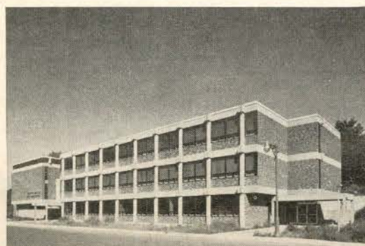
Beth Jacob School, Montreal. Archt: Schrier & Kessler. Genl. Contr: Montclair Construction Co. Ltd. Masonry Contr: A. Croteau & Fils Inc. Concrete & Precast Concrete Members: Francon Ltd.
