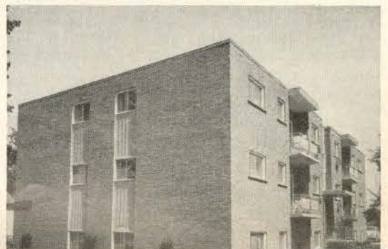
Apartment Building, Brantford, Ont. Owner & Builder: Galbar Investments Limited. Masonry Contr: Robert Poirier. Concrete Masonry Units: Brantford Brick Ltd. Ready-Mixed Concrete: Red-D-Mix Concrete Company.
