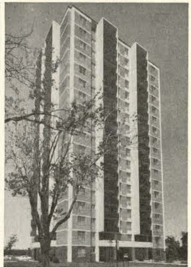
1000 Broadview Apartment Building, Toronto. Owner & Builder: Tova Developments Limited. Archt: Grozbord, King & Associates Ltd. Masonry Contr: Prime Construction Company. Concrete Blocks: Meteor Building Supplies Ltd. "Canada" Masonry Cement: Blair Supply Company Ltd.
