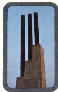
In most atmospheres Stelcoloy develops a tightly grained, closely adhering protective coating.
