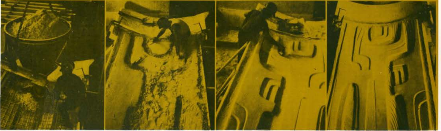
Working on the roughened 10 ft. x 8 ft. recessed area, sculptors apply wet cement over reinforcing mesh, adding finish with brush and trowel.
