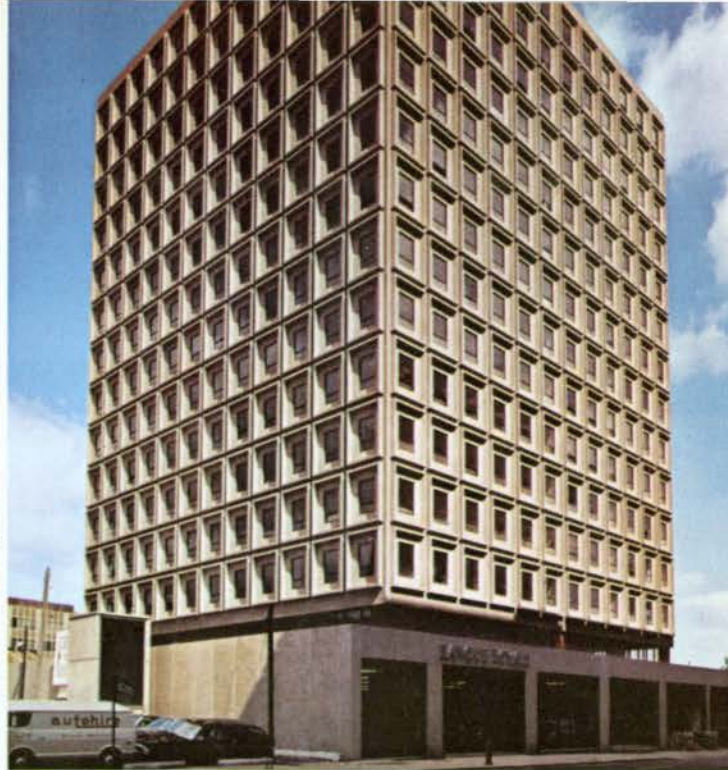
5 Precast concrete panels for the President Kennedy Office Building, Montreal.
