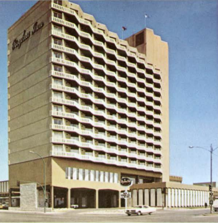
1 The Regina Inn, Regina, Sask., a modern, all-concrete building.
