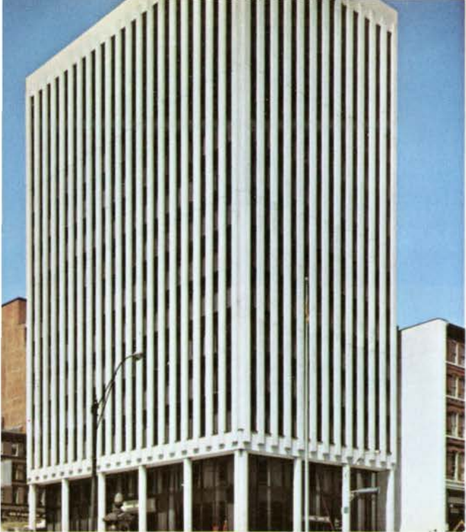
4 Brunswick House, Saint John, N.B., features precast concrete construction.
