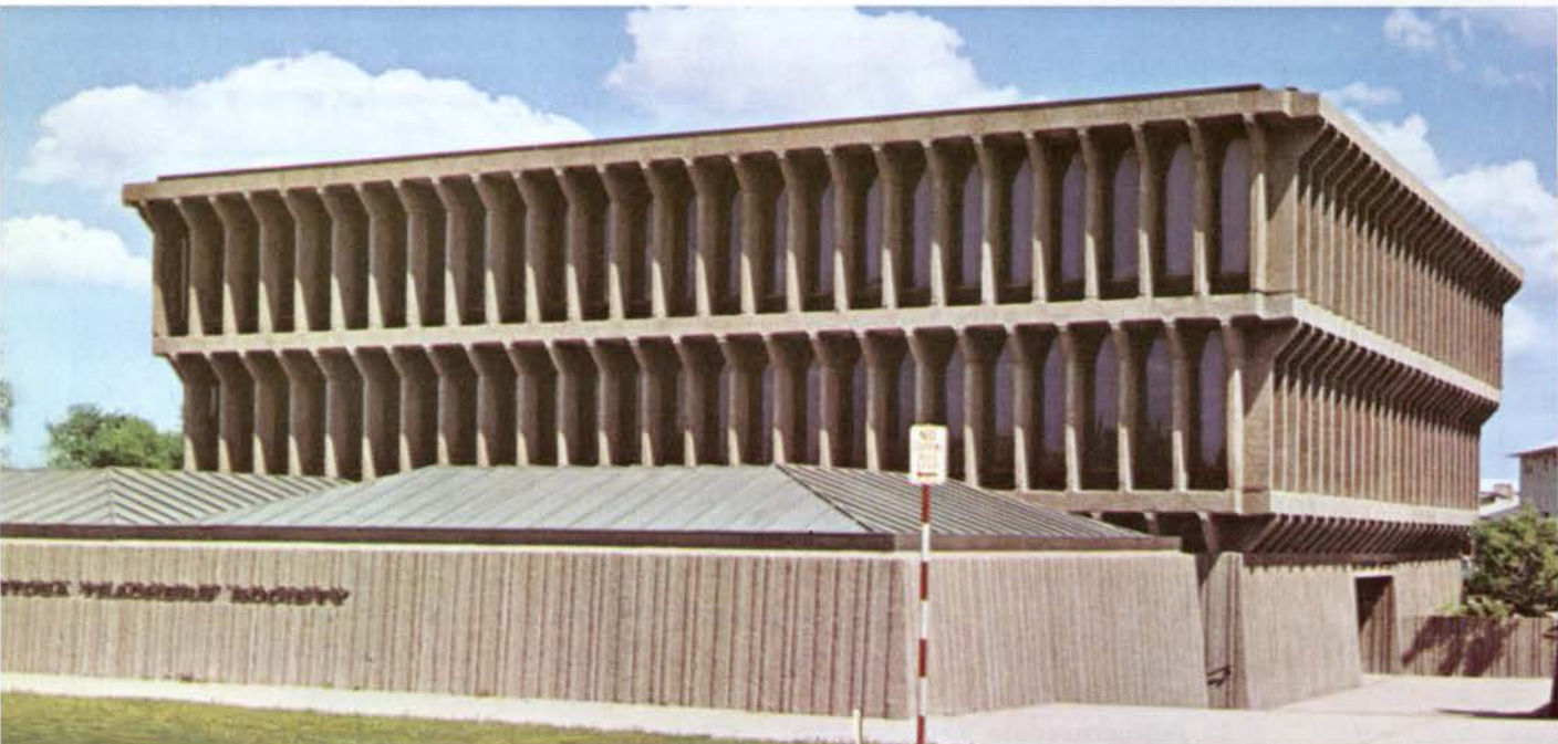
3 Headquarters of The Manitoba Teachers Society, Winnipeg, winner of the Manitoba Association of Architects 1968 Award of Excellence.
