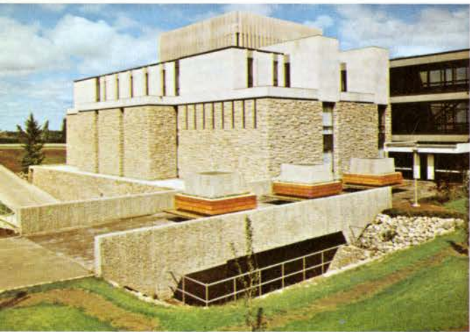
3 Precast concrete pedestrian bridge at University of Saskatchewan.
