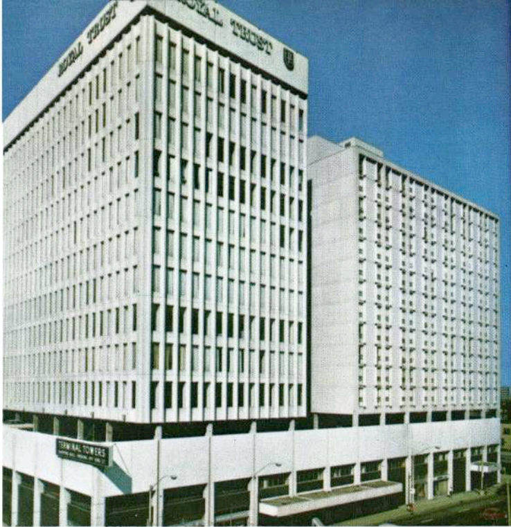
1. The Terminal Towers, Hamilton, Ont., features precast concrete panels.
