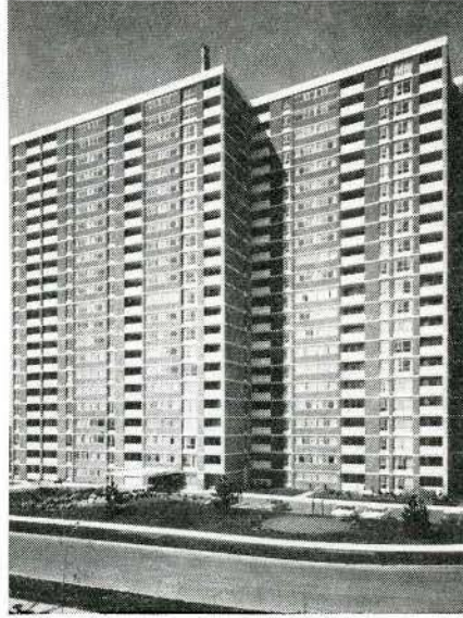
"Top of the Valley" Apartment Complex, Toronto, Ont. Owners: The Rubin Corporation & Mr. Jos. Godfrey. Architects: Henry Fliess. Consulting Structural Engineers: Reicher Bradstock & Associates Ltd. General Contractor: The Top of the Valley Limited. Masonry Contractor: Zachary De Vuono. Concrete Masonry Blocks: Richvale Block Supply Co. Ltd. Ready-Mixed Concrete: S. McCord & Co. Ltd.
