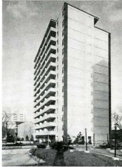
Gramercy House, Toronto, Ont. Owners & Builders: Greenwin Construction Company Ltd. Architects: Harry B. Kohl. Consulting Structural Engineers: Kazmar Consultants Ltd. Masonry Contractor: New Hillmount Construction Company. Concrete Masonry Units: Richvale Block Supply Co. Ltd. Ready-Mixed Concrete: Richvale Ready Mix Ltd.
