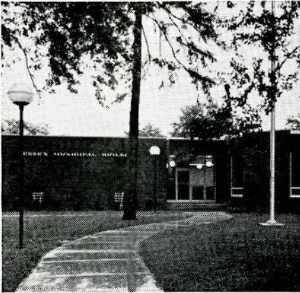
Essex Municipal Building, set among trees on the main street.
