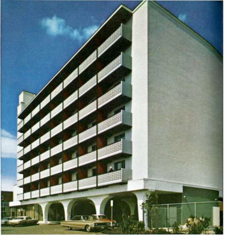
2. A variety of concrete masonry units for the Riviera Motor Hotel, Edmonton, Alta.
