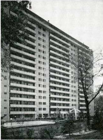
High Park Gardens, Toronto, Ont. Owners & Builders: Oak Pacific Holdings Ltd. Architects & Consulting Structural Engineers: Grozbord, King & Assocs. Ltd. Masonry Contractor: O. M. Construction Co. Concrete Masonry Units: Richvale Block Supply Co. Ltd. Ready-Mixed Concrete: Richvale Ready Mix Ltd.
