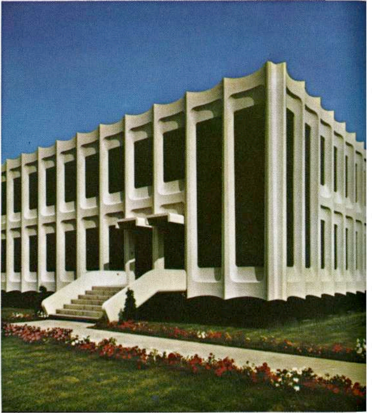
6. The Rodighiero Building near Montreal, a modern all-precast concrete building
