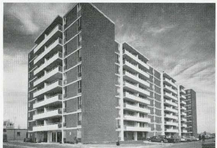
Prague Towers, 737 Birchmount Road, Toronto, Ont. Architects: Keywan & Kassian. Consulting Structural Engineers: Farkas, Barron, Jablonsky. General Contractor: Prague Towers Investment Ltd. (Owner & Builder). Masonry Contractor: Gottardo Contracting Co. Ltd. Concrete Masonry Units: Richvale Block Supply Co. Ltd. Ready-Mixed Concrete: Richvale Ready Mix Ltd.
