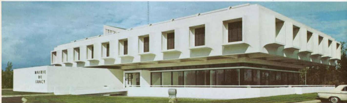
4. Imaginatively designed concrete panels provide unusual beauty and flawless uniformity for the City Hall, Tracy, Que.
