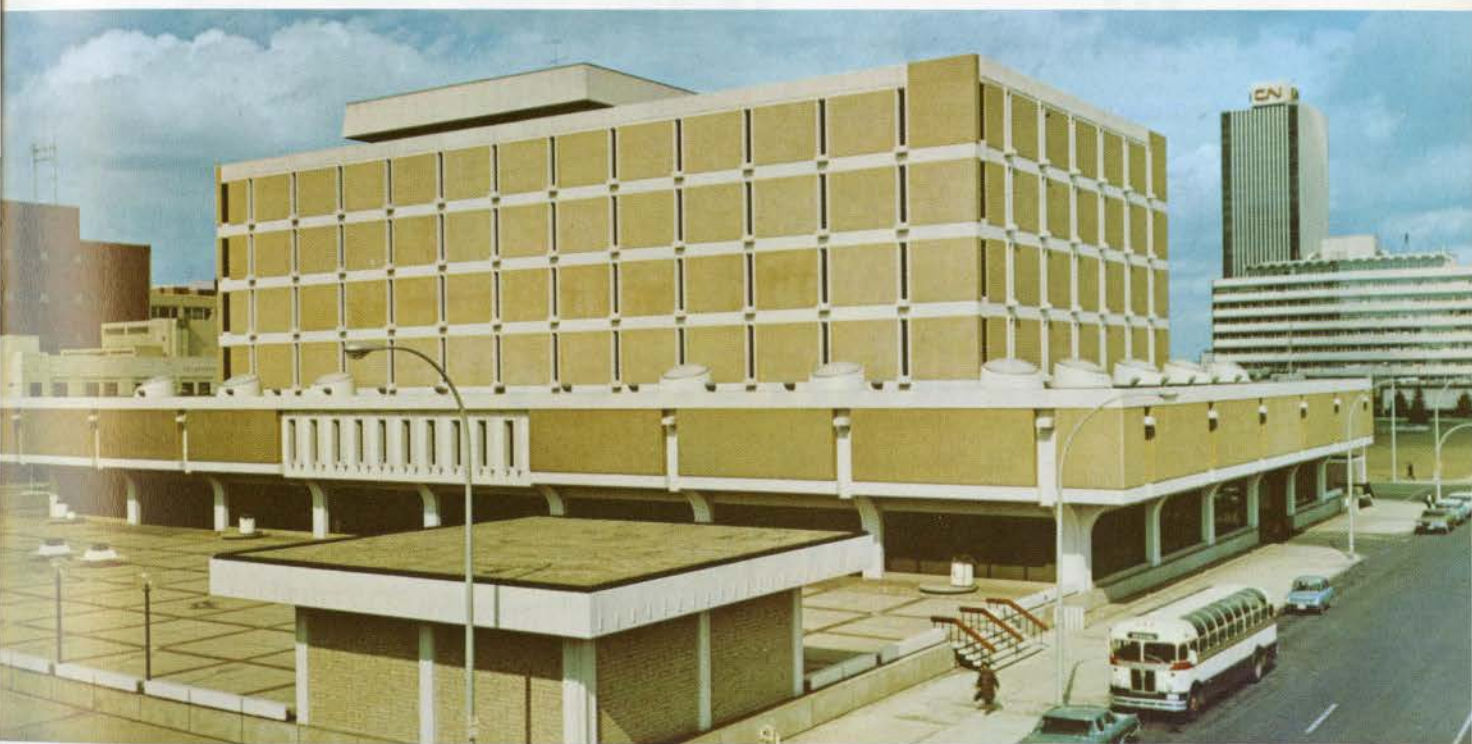
7. The Edmonton Centennial Library, a fine example of precast concrete construction. The CN Tower can be seen in background.
