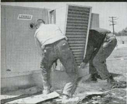
Optional POWER SAVER™ cools free with outside air below 57°F.
