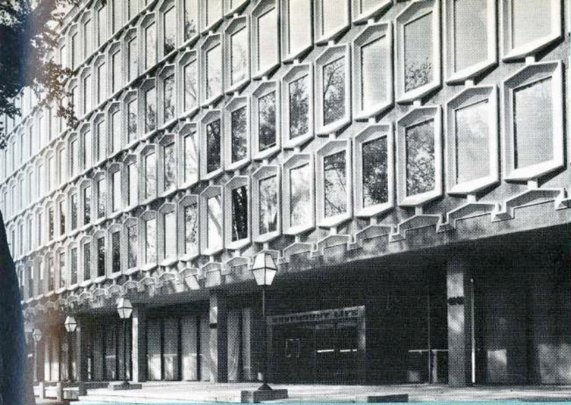
WESTMOUNT LIFE BUILDING. This is another application of Float glass by David Bloom of Montreal who was the first user of the product in Canada. The windows are set in precast concrete openings. Special metal frames for this project were developed by Pilkington who also did all the ground floor glazing. Owner/Contractors: David Bloom & Co. Inc. Architects: Kahn & Katansky.
