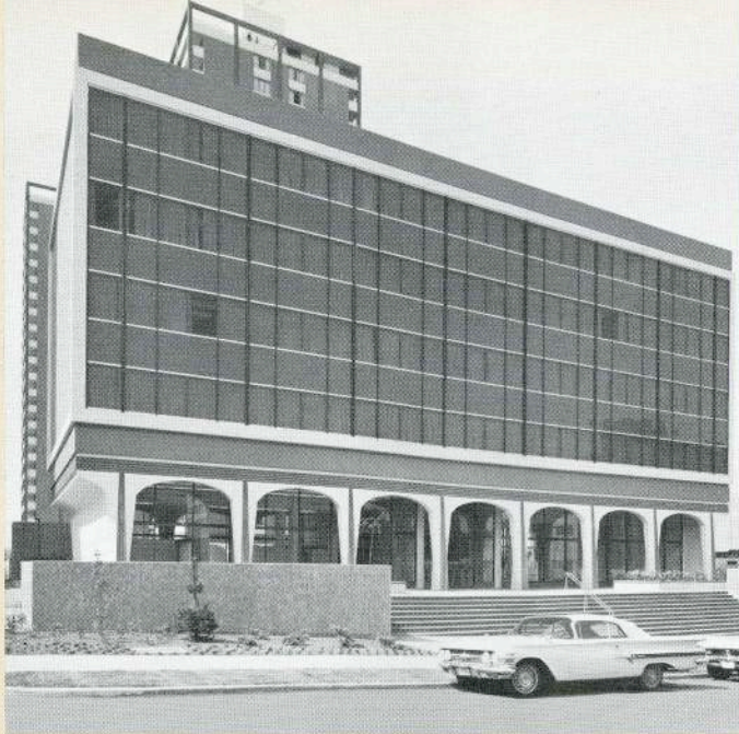
PACIFIC PALISADES OFFICE BUILDING—VANCOUVER. The curtain wall on this new building was a Pilkington project with all materials supplied and installed. The finish of the architectural metal is Permanodic. Other products include ¼" and ⅜" Colorclad, grey sheet glass and ¼" Float glass. Architects: B. Marr & Associates. Contractors: Zajac Construction.
