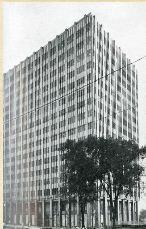
IMPERIAL LIFE—TORONTO. A custom curtain wall, it has a light bronze Permanodic finish with bronze insulating glass units. This is an excellent example of integral colour finish on aluminum. The ground floor has ⅜" plate glass in custom store fronts. Owner/Contractor: Yolles and Rotenberg Ltd. Architects: Webb, Zerafa, Menkes.
