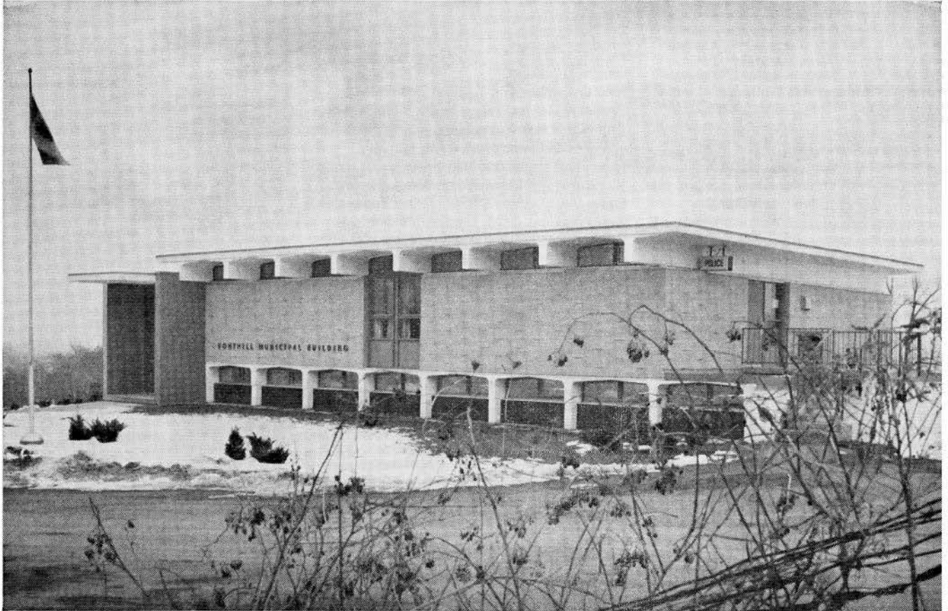
Fonthill Municipal Building, Fonthill, Ontario • Architects — Fraser & Macie, Welland. Consulting Engineers — Howard C. L. Joe & Associates, St. Catharines.
