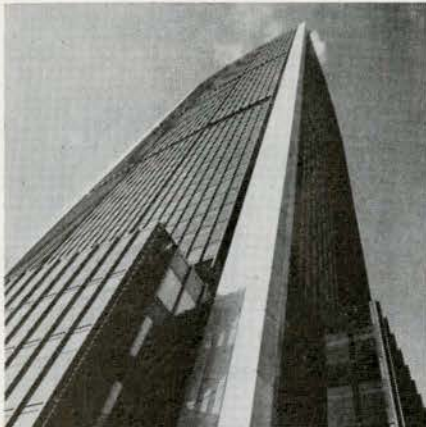
Place Victoria Stock Exchange Tower
