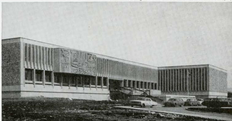
Bishop Grandin Academic Vocational High School, Calgary, Alberta Architect & Engineer: Cohos-Delesalle & Associates, Calgary
