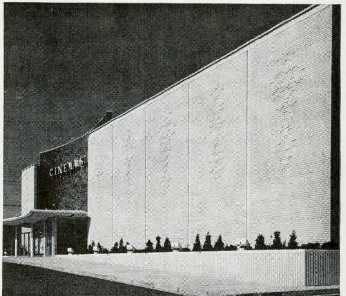
Les Cinémas Ste Foy, Que. Architects: Eliasoph & Berkowitz. General Contractor: Ain & Zakuta Ltd. Masonry Contractor: Victor Parent Inc.
