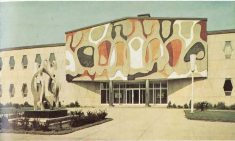
Painted concrete masonry walls at Western Warehouse Distributors, Calgary.
