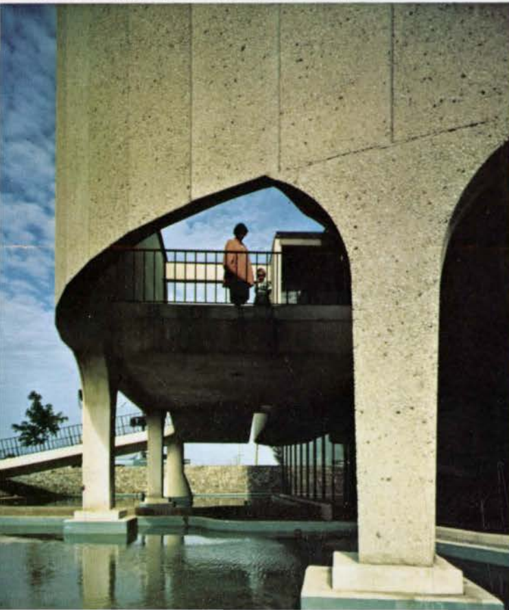
5 Exposed aggregate panels at the Duty-Free Building, Niagara Falls, Ont.
