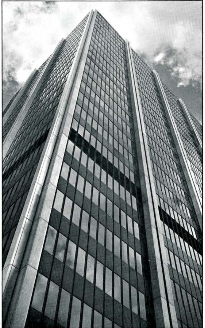
The new Richmond-Adelaide Centre, Toronto. A beautiful example of a complete curtain wall project.
