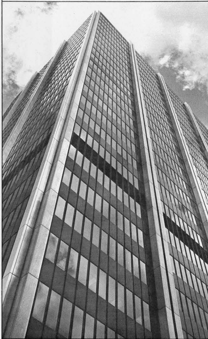
The new Richmond-Adelaide Centre, Toronto. A beautiful example of a complete curtain wall project.
