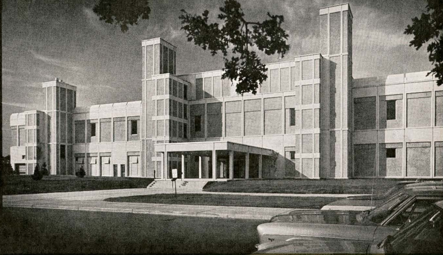
MO-SAI STRUCTURAL LOAD BEARING WALL PANELS, NORTHERN ELECTRIC ADVANCED DEVICES CENTRE, OTTAWA
