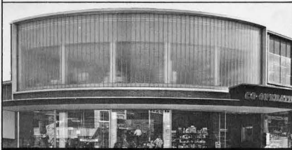
The curved elevation on the second story of this building is glazed with Profilit Glass.
