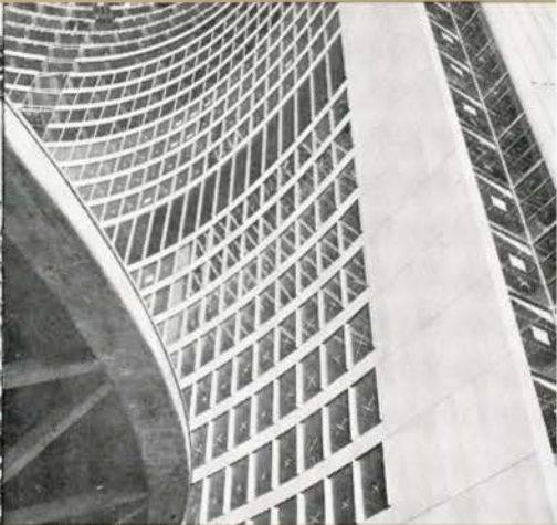
Spandrel and wall panels
