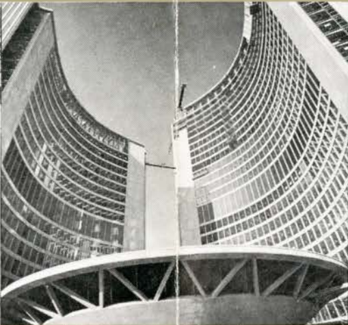
Precast struts on council chamber
