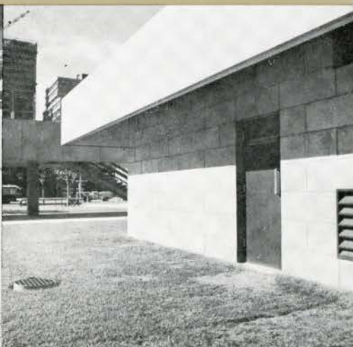
Pool house wall panels and fascia
