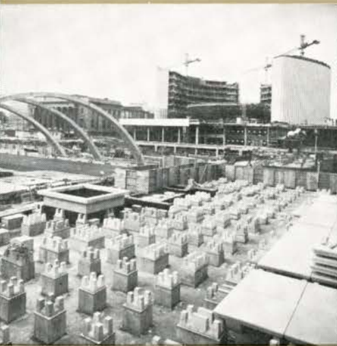
Precast pedestals supporting paving
