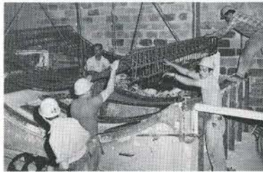
Precast Panel being cast
