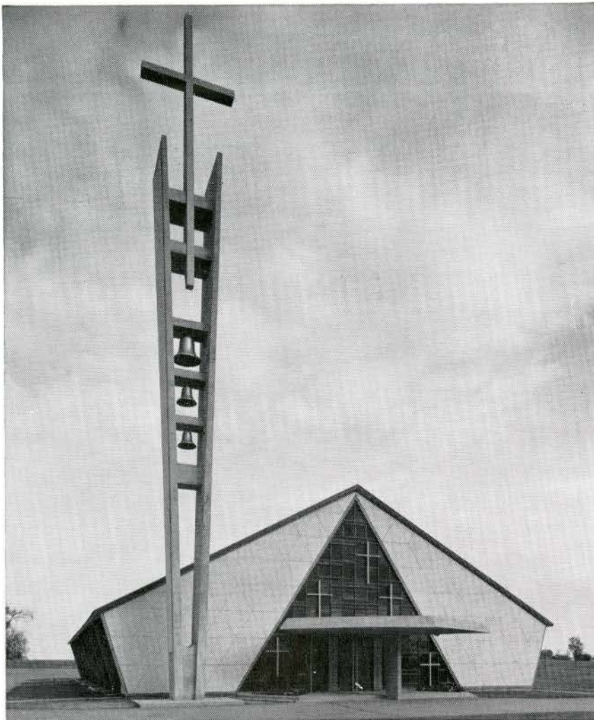
Our Lady Queen of the World Church, Richmond Hill, Ont. Architect: Gilleland & Janiss Architects' Consulting Structural Engineer: McNamara Engineering Limited. General Contractor: Perwin Construction Company Limited. Ready-Mix Supplier: Dual Mixed Concrete & Materials Company. POZZOLITH concrete was specified and used in the church and in the pre-cast Bell Tower. Master Builders EMBECO Non-Shrink Grout was used to grout the Bell Tower.
