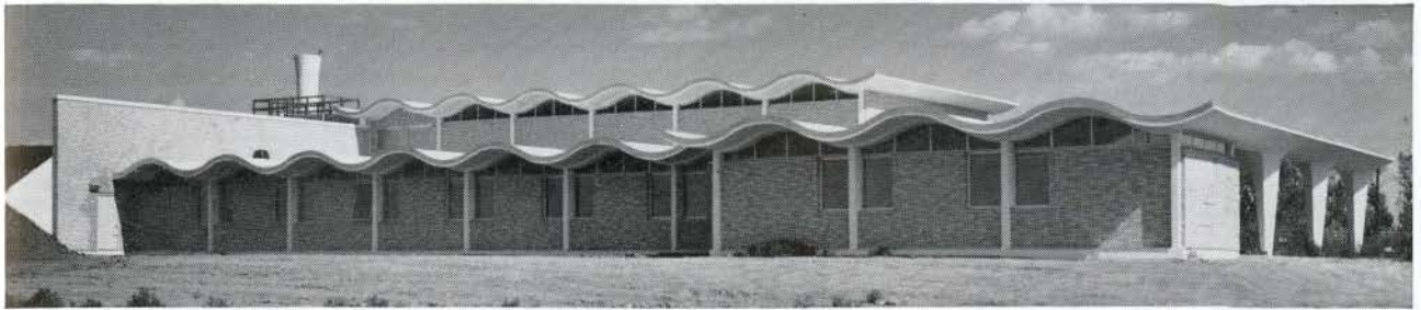
Linear Accelerator Building, University of Saskatchewan, Saskatoon, Sask. Architect: Tinos Kortes. Consulting Structural Engineers: Underwood, McLellan & Associates Ltd. General Contractor: Poole Construction Co. Ltd. Ready-mixed concrete supplied by: Stodola Concrete (Sask.) Ltd.
