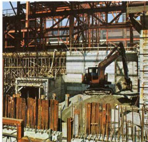
View over scale pit into slab furnace area.
