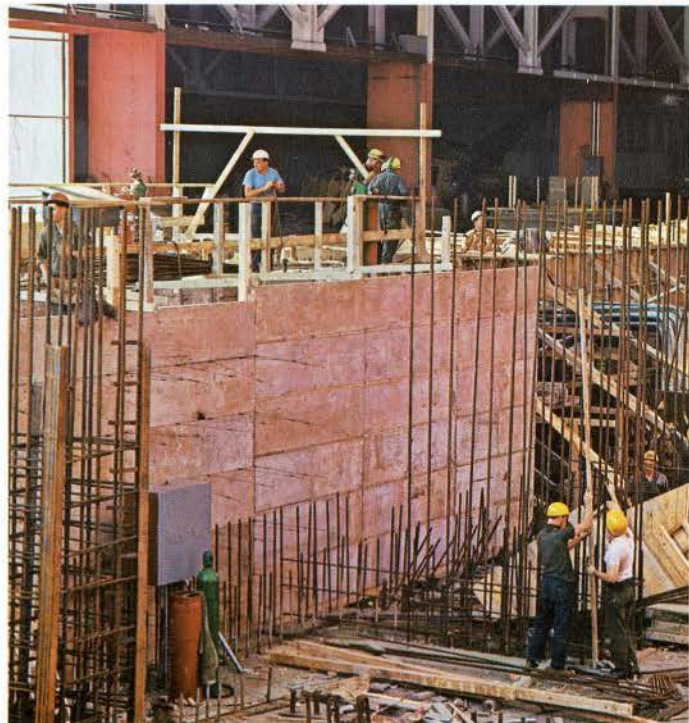
Reinforcing steel and formwork for equipment foundations.
