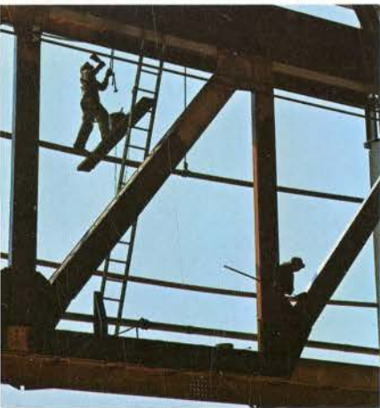
Portion of truss to carry crane rail.
