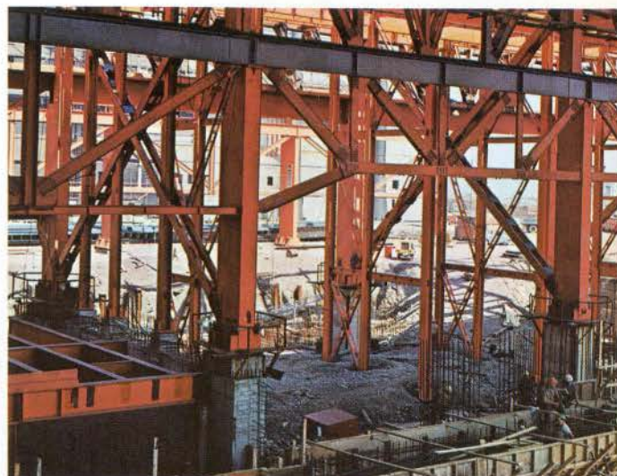
Structural steel for building to house slab furnaces.
