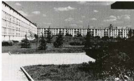
Prefabrication applied to large scale housing Sarcelles, Paris
