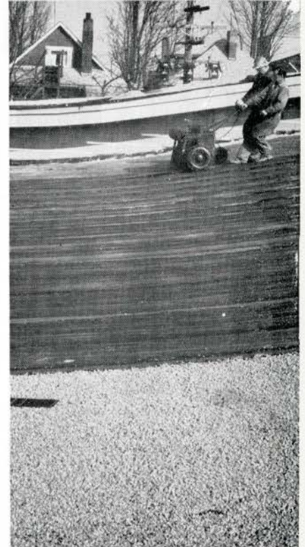
Flexible Fir Plywood panels nail easily to joists on gently curving roofs. Light weight structure utilizes 2" rigid insulation under built-up roof. Vancouver, B.C. Safeway Store. Architect - F. E. Roy.
