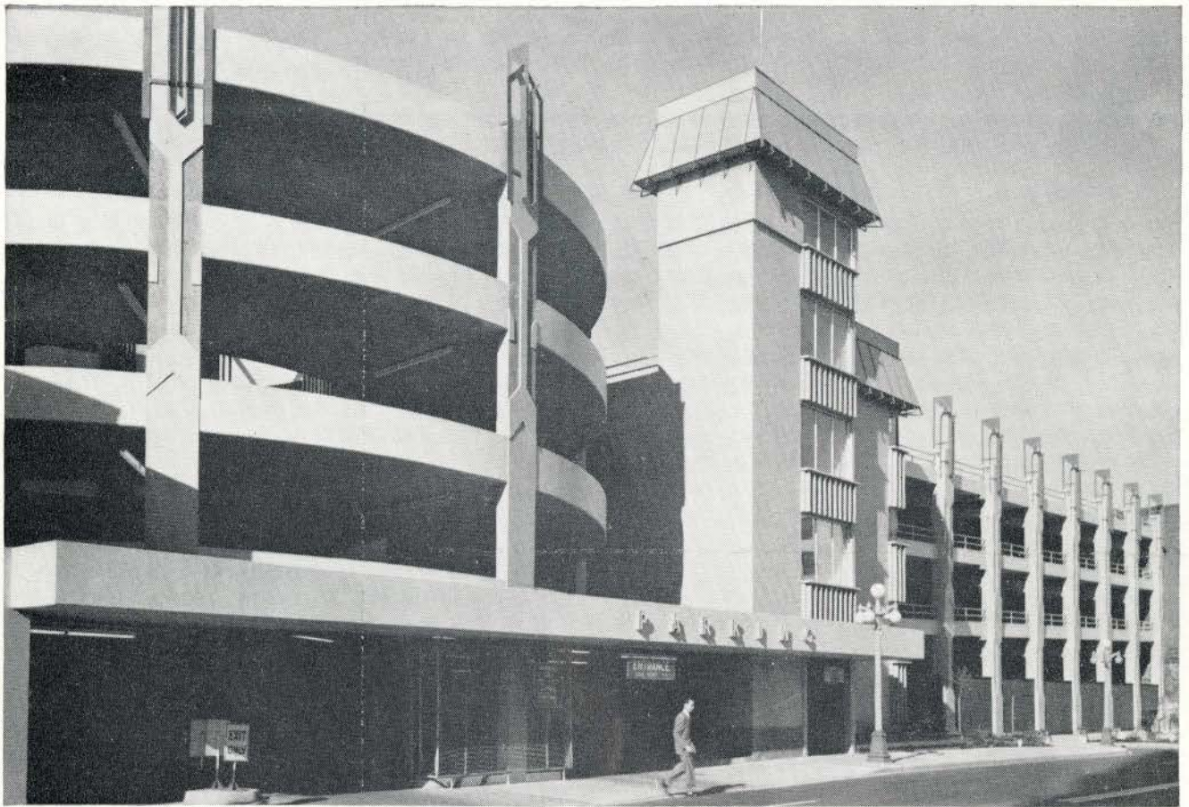
View Street Parkade Garage, Victoria, B.C. Architect: John A. DiCatri. Engineer: A. B. Sanderson & Co. General Contractor: Farmer Construction Ltd. Ready Mix Supplier: Ocean Cement Ltd.
