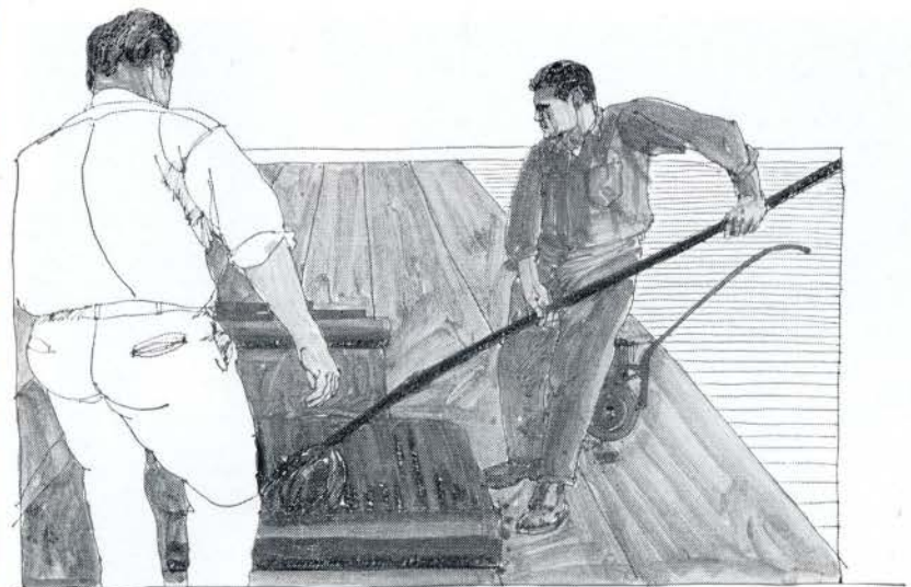
Felt being mopped over factory-coated base sheet. Hot asphalt does not contact Roofmate FR.
