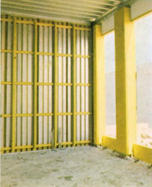
(Above) Each pair of columns with transverse members enclose a window frame.
