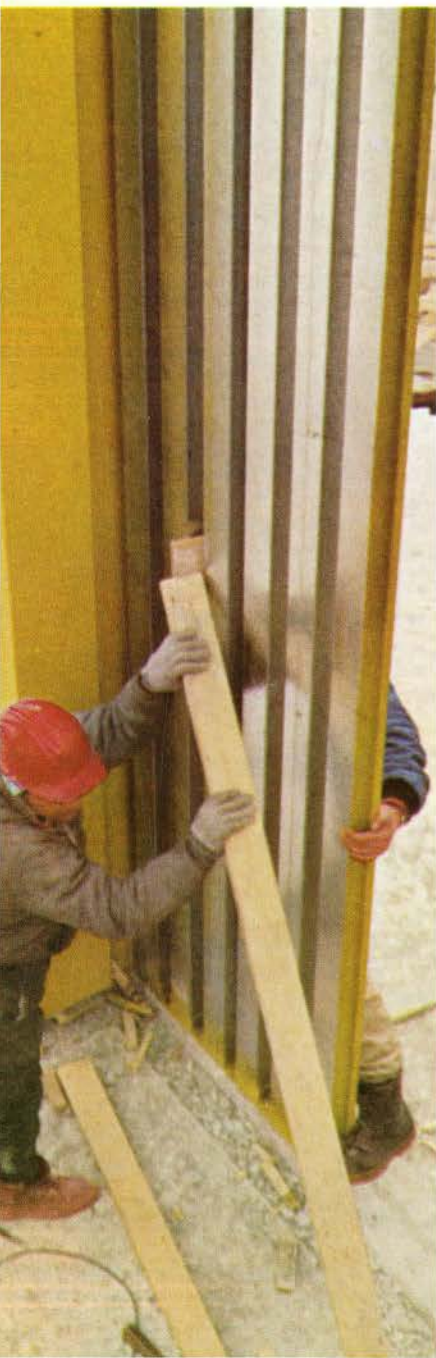
(Above) Each pair of columns with transverse members enclose a window frame.
