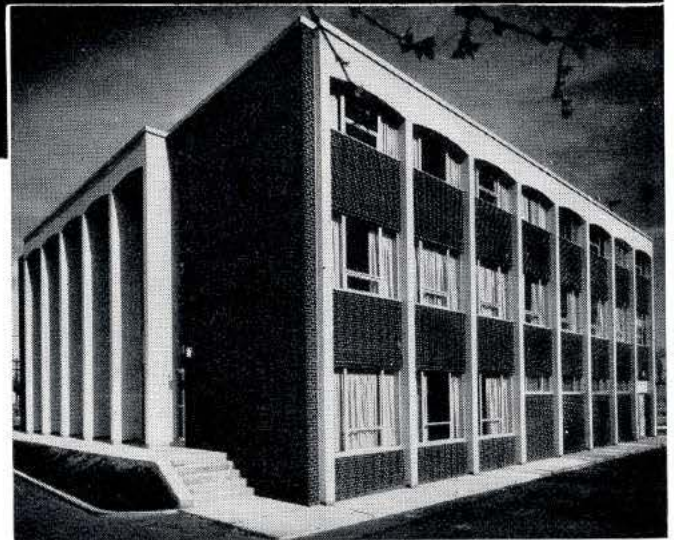
ARCHITECT: Sproatt and Rolph MAGISTRATES COURT BUILDING, Willowdale, Ont. GEN. CONTR.: Stowe and Gould Ltd. PRECAST PANELS BY: Pre-Con Murray Ltd.
