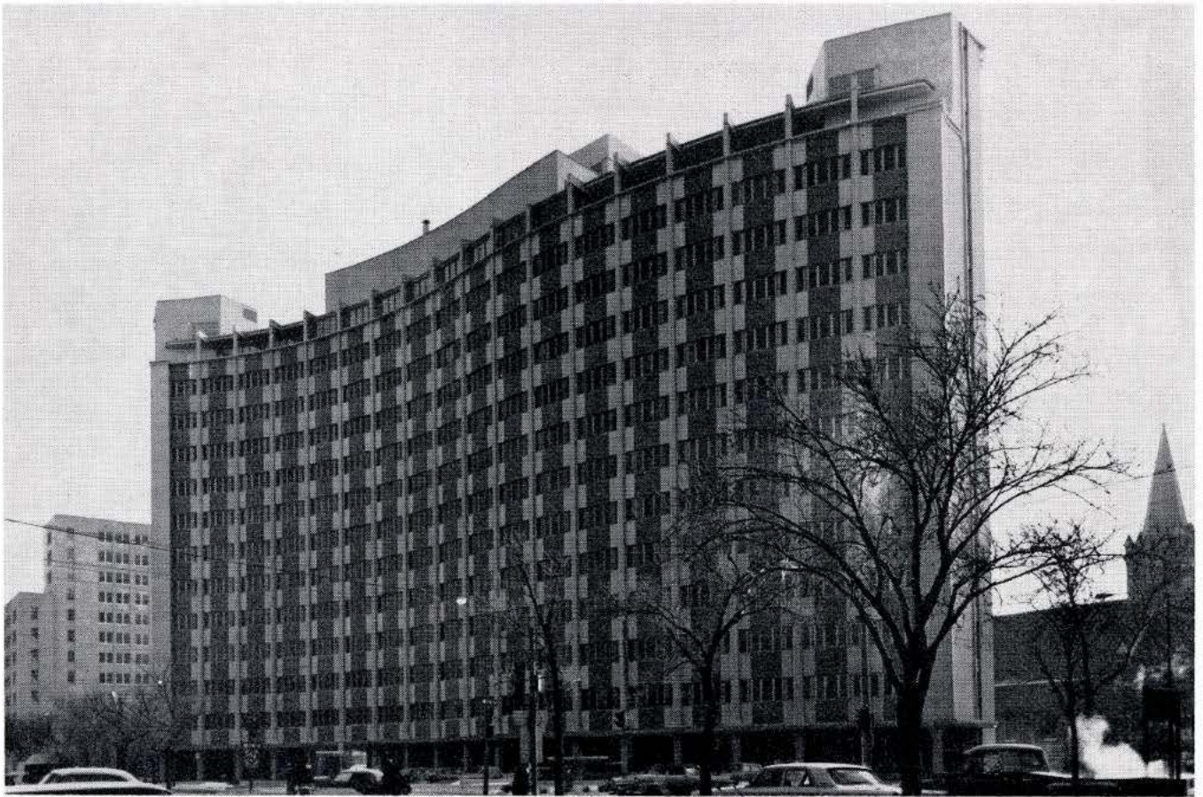
Saskatchewan Power Corporation Building, Regina, Sask. Architect: J. Pettick, MRAIC.
