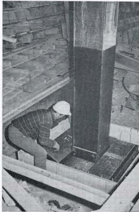
Installing lead-asbestos anti-vibration pads on top of column base plate
