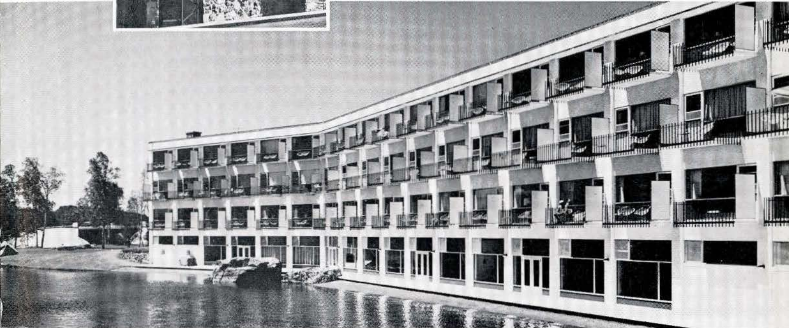
HOTEL L'ESTEREL, Ville d'Esterele, P.Q.; Architect: Jean-Guy Clement; Contractor: Simard et Freres Cie. Ltee. Rotary Oildraulic Elevator sold and installed by Alpin Elevator Co., Ltd., Montreal, P.Q.
