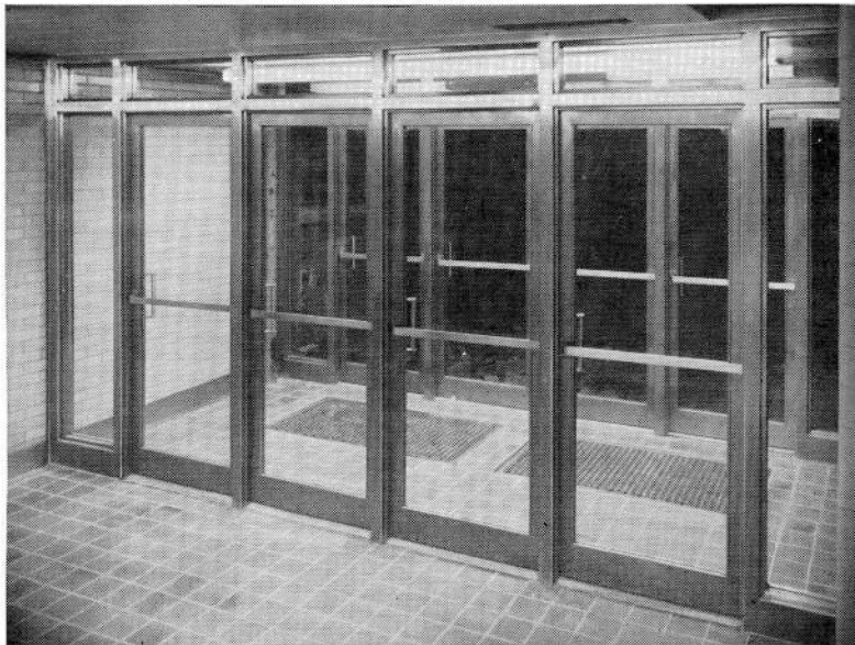
Entrance to TCA's service building at Dorval Airport, Montreal. Owner: Department of Transport. Architect: W. Ramsay. Associate Architects: Illsley-Templeton-Archibald Larose & Larose General Contractor: Foundation Company of Canada Limited.
