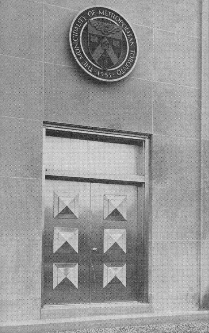
Front doors, Eglinton Reservoir station, Toronto. Designed by Gore & Storrie, Ltd.
