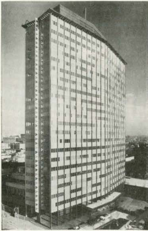
B.C. ELECTRIC CO. LTD. —Architects: Sharp, Thompson, Berwick & Pratt General Contractor: John Laing & Son (Canada) Ltd.
