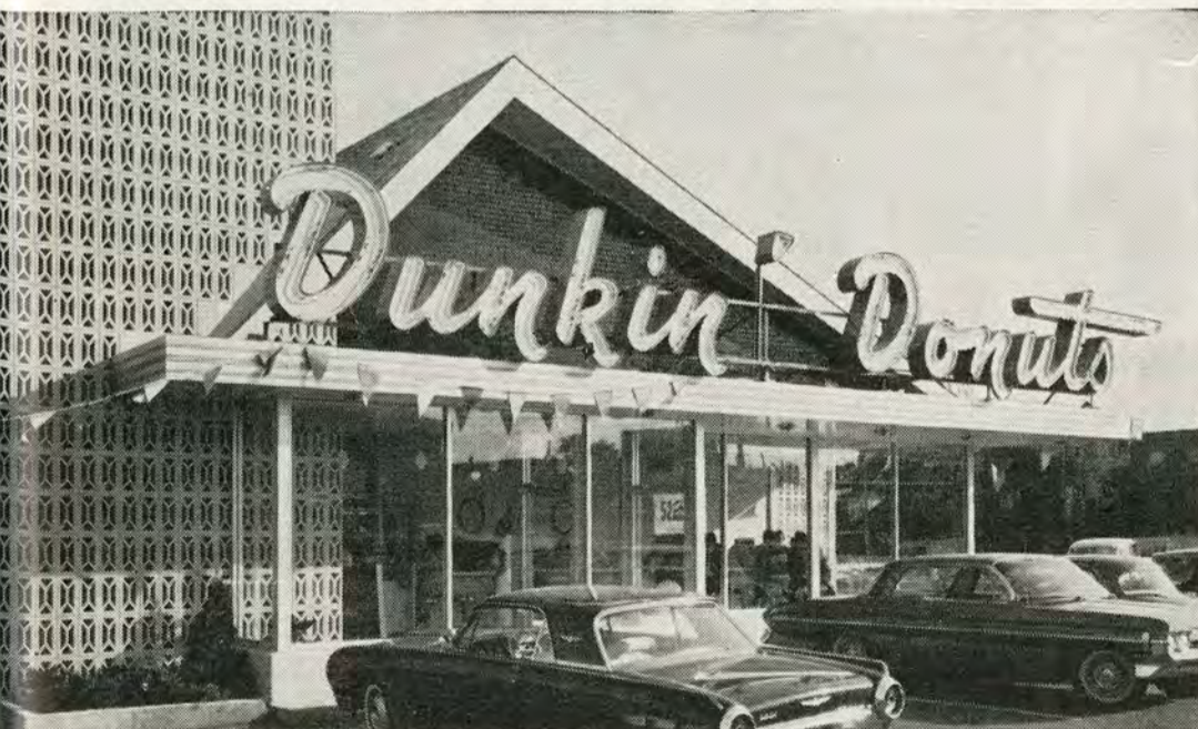
DUNKIN' DONUTS RESTAURANT , Montreal. General Contractor: Lincoln Construction Inc. , Montreal. Concrete blocks supplied by H. Beaudry Concrete Blocks Co. Ltd. , Montreal.
