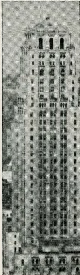
Canadian Imperial Bank of Commerce Building
