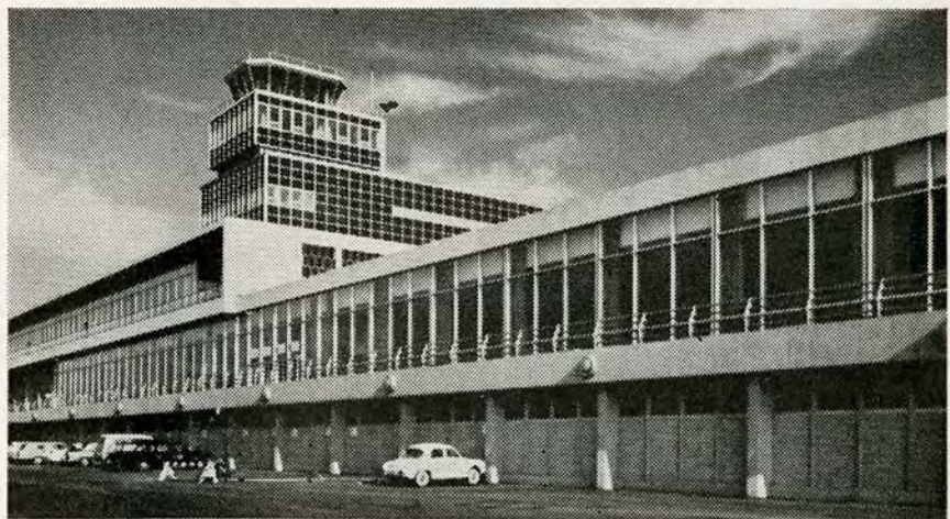
Twindow installation at Montreal International Airport, Dorval, P.Q. ARCHITECTS: Illsley, Templeton & Archibald, Larose & Larose, Associated Architects GENERAL CONTRACTOR: The Foundation Company of Canada Limited GLAZING CONTRACTOR: Canadian Pittsburgh Industries Limited
