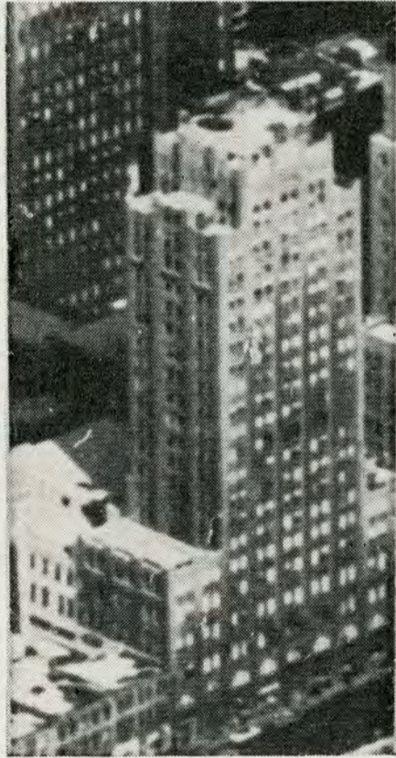
Stair Building Star Building
