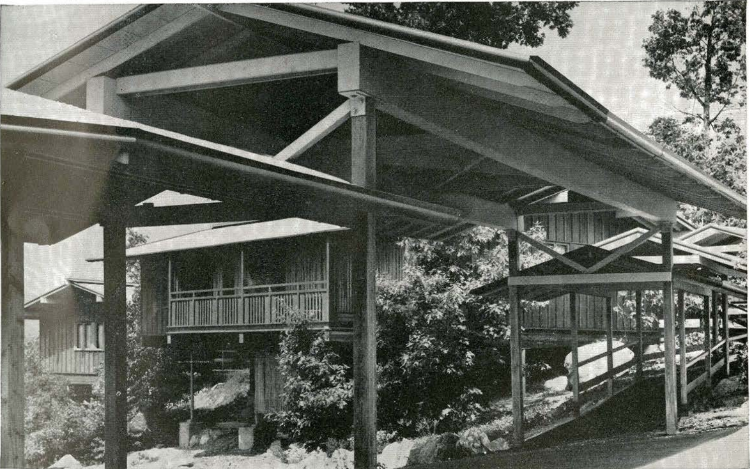
The rugged strength of exposed framing, the durability of planked roofing and board-and-batten siding are used to advantage in this complex of wood structures.
