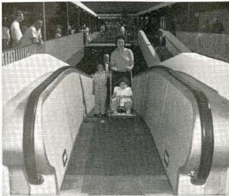
Large shopping centre uses Speedramp to carry people from parking area to central mall area.
