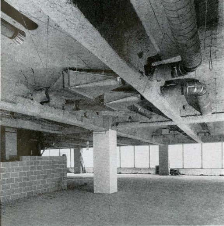
Air conditioning ducts go through the steel beams.
