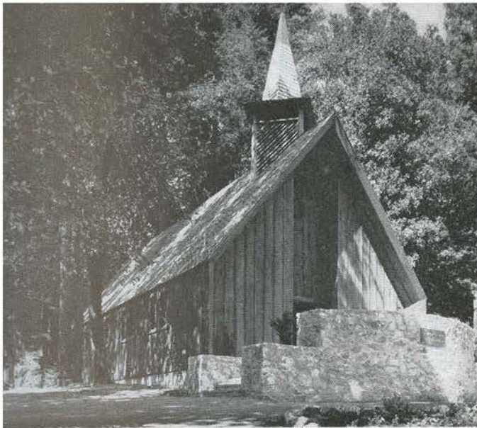
A chapel in the woods sets simply, reverently in its site with the natural belonging of board-and-batten siding, shingled roofing, and a louvered wood steeple.
