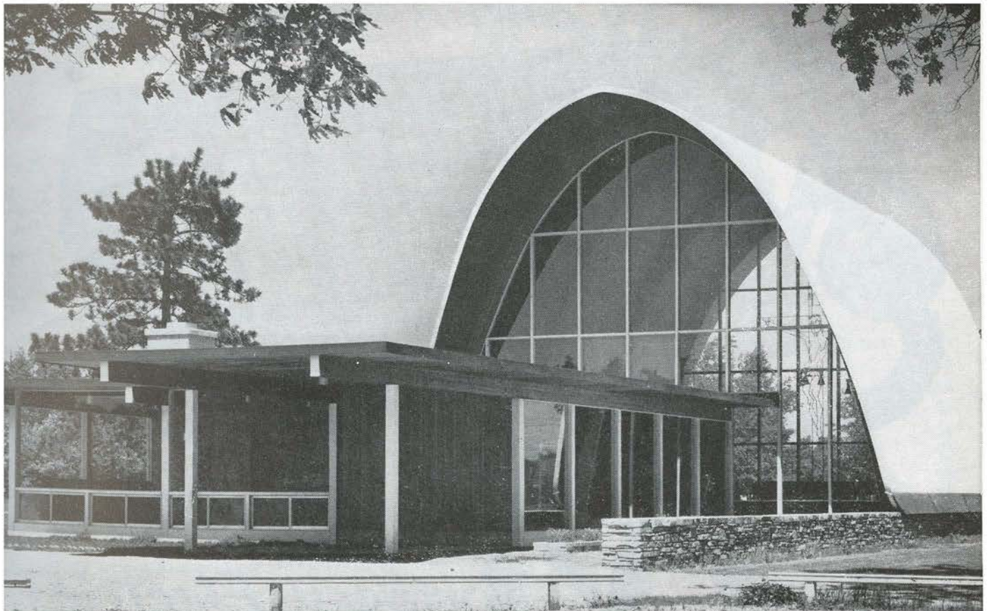
Gracefully bowed laminated beams supporting a parabolic arch, spacious wood-framed glass areas at either end—all combine to create a wide-open setting for a unique treatment of the crucifix. Note how simplicity of design dramatically demonstrates wood's quality throughout this unusual house of worship.
