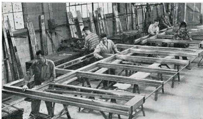
Chubb Craftsmen weld the doors to form one complete unit
